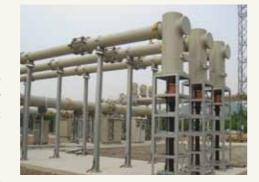
They also use epoxy insulating plate to isolate between cable sheath and GIS chamber. The SVLs(Sheath Voltage Limiter) can be installed to protect epoxy insulating plate from switching impulse. Upon request
